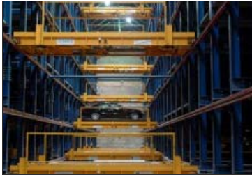
The robot car park can park 250 cars an hour
